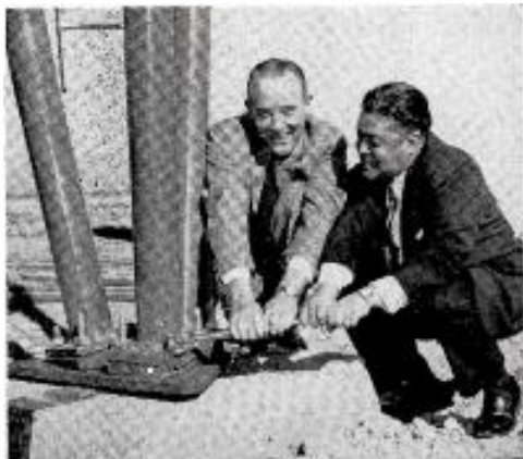
FINISHING TOUCHES to big bolts anchoring the 752-ft. transmitter tower of KOSA-TV Odessa, Tex., are put on by Cecil L. Trigg (l), president and general manager, and Paul Mowrey, New York television consultant. KOSA-TV, a CBS affiliate, began programming Jan. 1.
